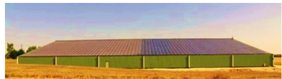
Figure 2: Twin generator of 250 kWh.
