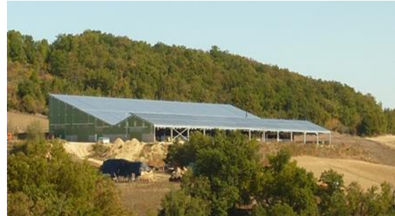
Figure 1: The demonstrator is located on the farm in Saint- Marcel . The photovoltaic plant has a power of 777 kWp for a surface of 7000 m 2 .
